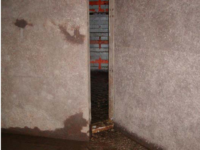
7) Entrance weir guides – same as above.
